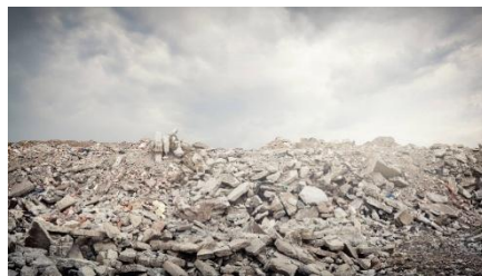
Figure 2: Construction and Demolished Wastage
